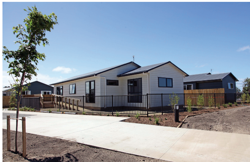
16 relocatable houses were moved onto the Guild Street site.
